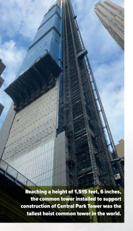
extraordinary access solution - installing the tallest hoist common tower and the largest continuous rack and pinion hoist in the world – which earned the company a SAIA Project of the Year award in the Masts Driven Hoists and Platforms category. Perhaps even more amazing is the fact that approximately 1,440 feet of the 1,515-footsix-inch common tower structure was partially cantilevered using massive steel dunnage.
