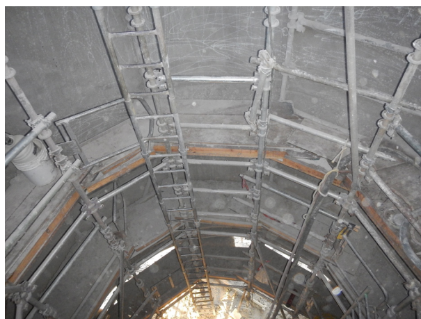
Figure 3. This scaffold provides access to a repaired FCCU regenerator where the dry gunning technique was used to install refractory.
