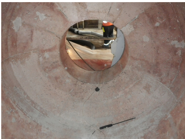
Figure 5. A field installed vibe cast of the air pre-heater.
