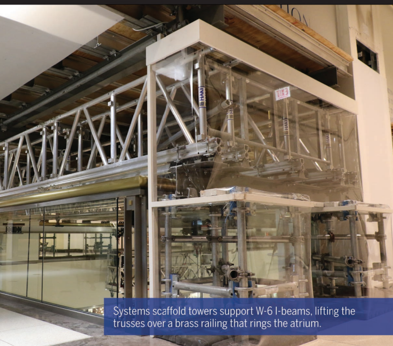
A custom-designed "shoe" connects the HAKI trusses to the steel header beams.
