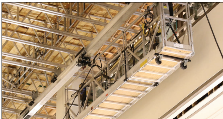
The ability to slide the suspended platform meant that renovation work on the fascia could proceed without interruptions for re-rigging.
